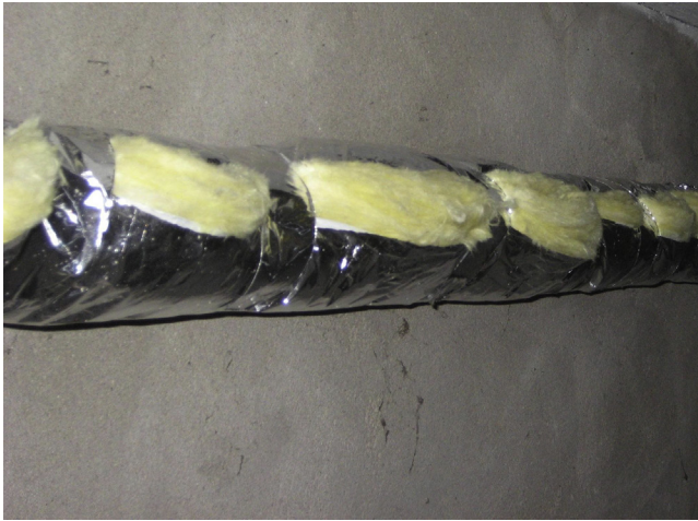
Figure 4.13 Fiberglass batting has already proven to be an excellent harborage of dust, insects, and rodents.
