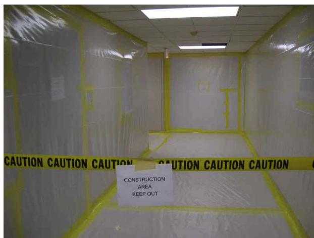
Figure 3.1 Cleanliness of ongoing process operations should be maintained by construction of temporary partitions and dust barriers. The construction side should be under negative pressure relative to areas with ongoing process operations. RenovationIMG_7846.
