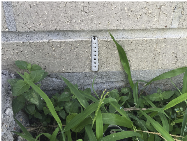
Figure 4.6 A cover prevents access of insects and rodents in the weep hole. Courtesy of Tamlyn – Connected to the Industry®.
