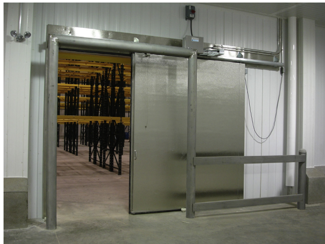
Figure 4.10 Horizontal sliding doors allow for hygienic operations, at the condition that all gaps are closed between the door and the frame with gaskets of rubber or bush stripes. Sliding doors should not have channel floor tracks. Protection of the door, door frame, and wall is required. Courtesy of The Stellar Group.
