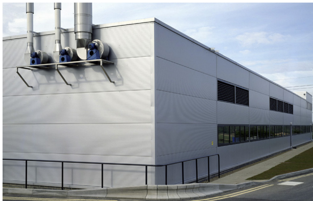
Figure 4.3 Areas in a perimeter of 3 m of the factory must be kept free of vegetation to avoid pest breeding and harborage sites. There should be a gravel strip and path around the factory building of at least 90 cm. No shrubs or plants should be located in the close vicinity of the factory building (Moerman, 2010).
