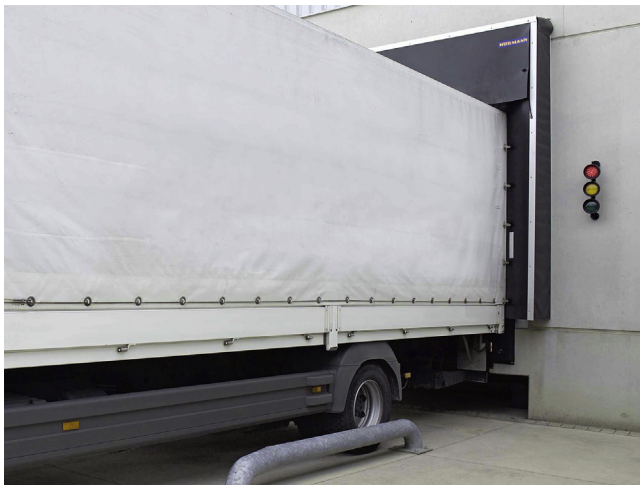
Figure 4.11 Dock shelters, such as canopies above, and dock-seal systems, such as cushion-closure seals around the truck doorways, will reduce the infiltration of warm, humid air and rain into refrigerated loading docks. These measures also prevent the entry of insects. Courtesy of Hörmann KG.
