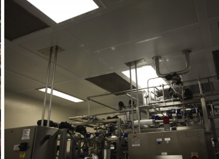
Figure 4.48 (a) Uncluttered ceiling with lighting having a sloped body with the lower part provided with a polycarbonate glass ( Courtesy of Veelite Technologies, Ltd. ). (b) Uncluttered ceiling. Lighting can be built in into the false ceiling with a hermetically closed seal and further separated with a transparent polycarbonate glass from the process area just below. It is a procedure typically for high hygiene areas where lamps are changed via the technical area ( Courtesy of Environmental Systems Corporation, ESC Cleanrooms (Moerman, 2011b) ).
