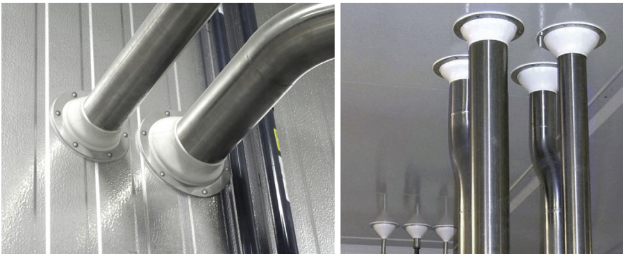
Figure 4.36 Pipetite is a silicone wall or ceiling boot which attaches to the wall or ceiling and forms a flexible seal around the pipe.
