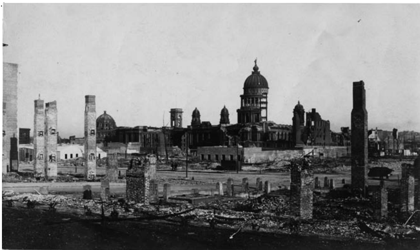
Figure 3.3 San Francisco's 1906 Earthquake: City Hall, April 1906. CHS 2009.123; FN-36064, SF-EQ (1906). Courtesy: California Historical Society, San Francisco, CA.
