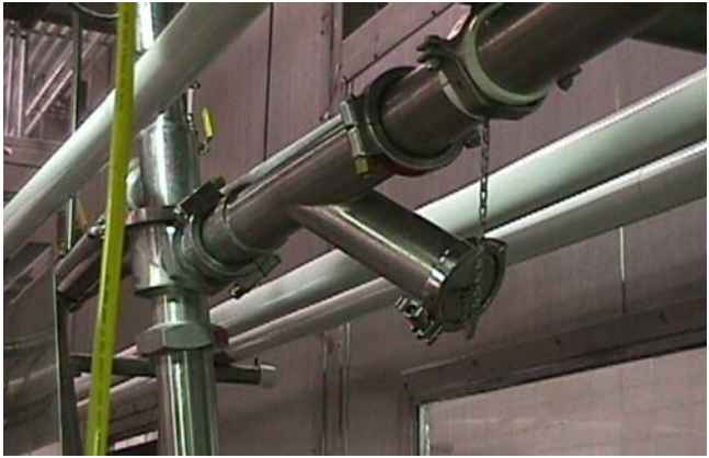
FIGURE 7.30 This drain point pointing downwards acts as a dead leg (organization Sanitary Design Workshop, © 2016).
