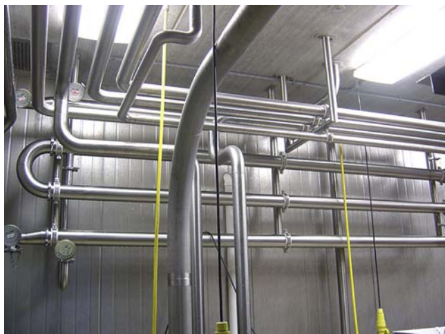
FIGURE 7.39 For suitable cleaning, process equipment and piping must be installed at sufficient distance off the wall, ceiling, and floor. Courtesy of CSI Central States Industrial, www.csi-designs.com .
