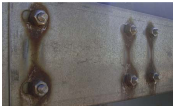
FIGURE 6.1 In this part of the food processing equipment, galvanized steel plate is combined with stainless steel bolts, giving rise to galvanic corrosion between the stainless and galvanized steel components.
