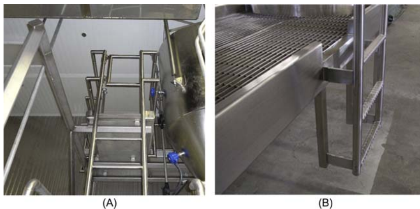
FIGURE 6.80 (A) The framework of the platform consists of closed square section members turned through 45 degrees (diamond configuration). The solid deck plates of the walkway are mounted a distance from these horizontal framework members. Kickplates are installed at the perimeter of the platform deck. Handrails and rungs of the ladder are made of round tubing (courtesy of The Stellar Group). (B) The ladder is installed about 200 mm above ground level. Because the ladder makes no floor contact, the factory floor below the ladder can be cleaned very easily. Ladder rungs are covered with nonslip surfaces. Open metal grid is used as decking, although not recommended, especially if food is passing beneath the platform. However, solid deck plates provide fewer niches for food debris to accumulate and microorganisms to grow, and they are also much easier to clean. Photo left, courtesy of The Stellar Group; photo right, courtesy of Bay State Industrial Welding & Fabrication, Inc.
