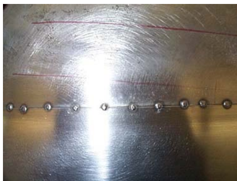
FIGURE 7.2 Spot welds create crevices and may retain product residues, as well as harbor microorganisms.
