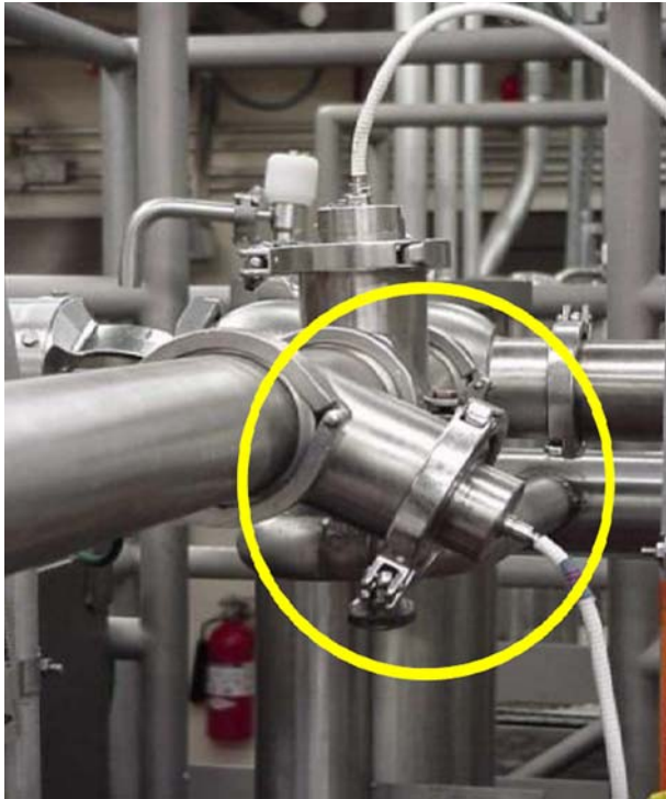
FIGURE 7.79 An instrument branch facing downward instead of inclined upwards creates a difficult-to-clean dead area where condensate, debris, suspended solid particles, flakes, etc. may accumulate. Fluid velocities in the dead leg are much lower, and thus the area of entrapment may not be reached by cleaning or sterilizing procedures, hence leading to contamination of the product. Courtesy of Joe Stout, Commercial Food Sanitation LLC - Intralox, © 2016.
