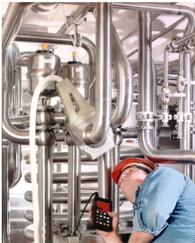
FIGURE 7.35 Stainless steel hygienic tubing joints should be made by automatic orbital welding where possible. Orbital welding provides smooth and crevice-free junctions (Kopitzke et al., 2006).
