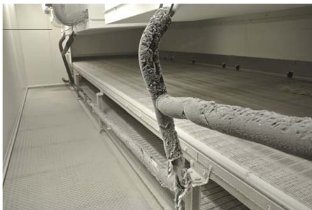
FIGURE 7.37 The cladding which surrounded the insulation of the refrigerant supply and removal piping was probably lost during high-pressure cleaning operations. Now, worn off particles of insulation may be entrained by the airflow into the product (Moerman & Fikiin, 2016).
