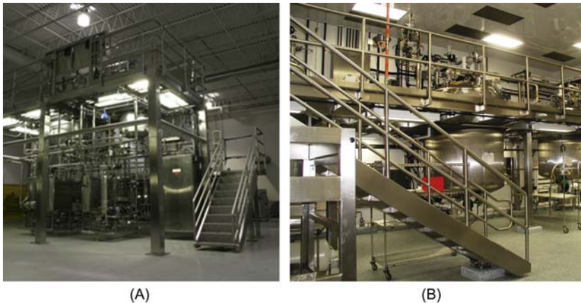
FIGURE 6.82 (A) Connecting the framework of stairs, walkways, or platforms to a floor usually occurs by means of a base plate securely fastened to the floor by means of a fixing bolt (courtesy of Holland Applied Technologies). (B) Base plates also can be fixed to a floor plinth, thus prohibiting dirt and liquids from getting under the base plate during process and cleaning operations. The stringers of staircases make no floor contact, hence facilitating the cleaning of the factory floor. Photo left, courtesy of Holland Applied Technologies; photo right, courtesy of Bay State Industrial Welding & Fabrication, Inc.)
