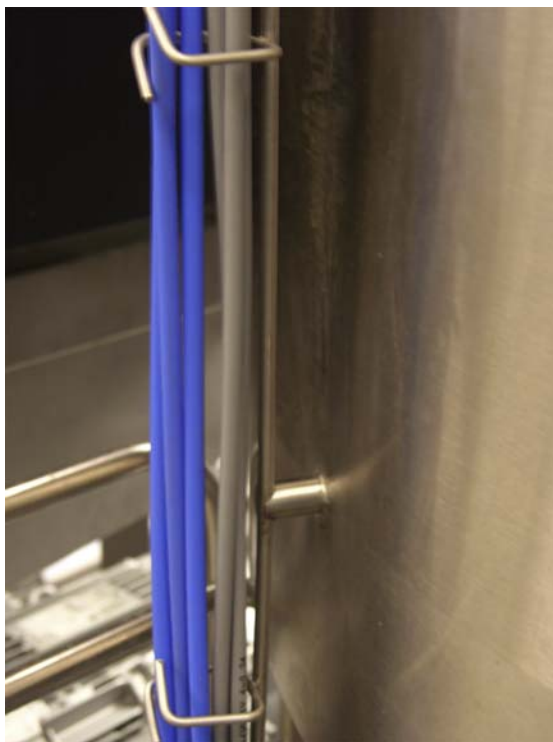
FIGURE 6.73 Cable support system with a minimum number of members. The number of loosely fixed cables should be minimal, to avoid uncleanable entangled cable arrangements.
