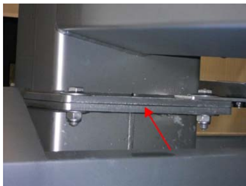
FIGURE 8.21 Metal-to-metal sandwiched area giving rise to a crevice where microorganisms may establish a niche to grow and the framework may rust. Courtesy of Joe Stout, Commercial Food Sanitation LLC - Intralox, © 2016.
