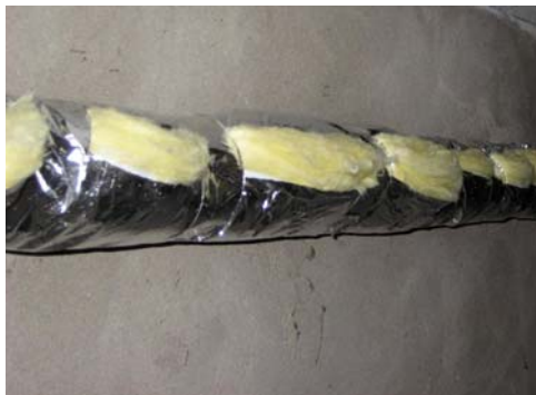
FIGURE 7.36 Fiberglass batting has been proven to be an excellent harborage of dust, insects and rodents (Moerman & Wouters, 2015).
