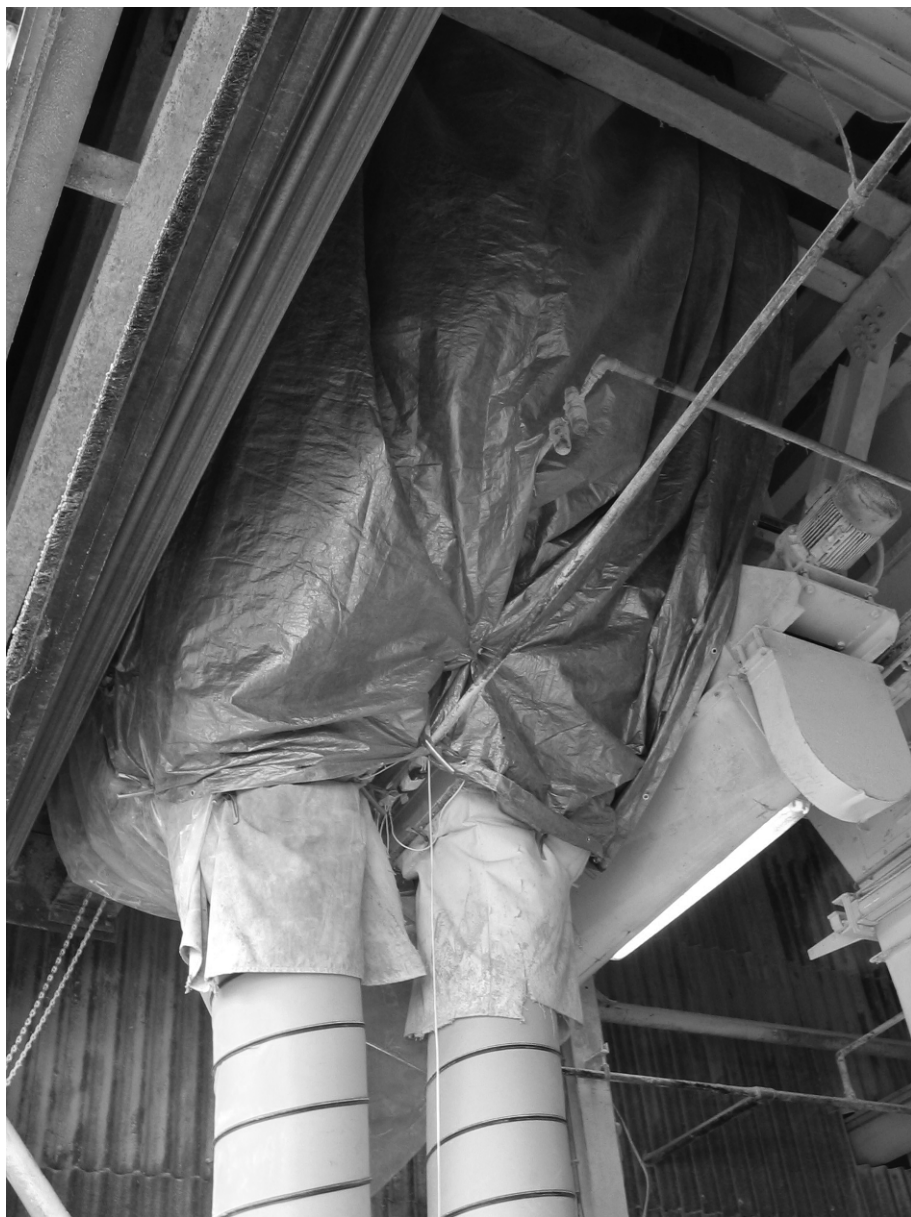
Figure 5.2 Access point for heat treatment of a silo.
