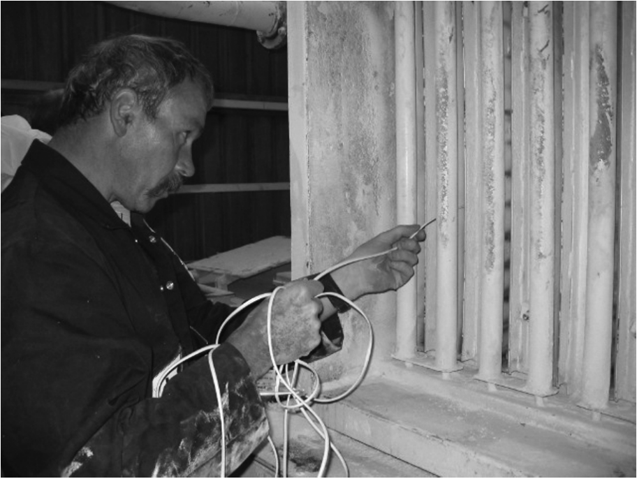
Figure 4.4 Heat sensor to monitor heat treatment of food machinery.
